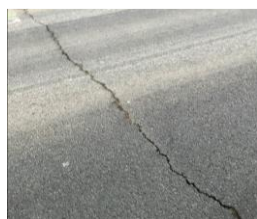
Fissure Transversale
