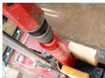
Figure II-15. Sample coring
