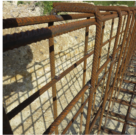
Figure 4-47: Welded reinforcement.
