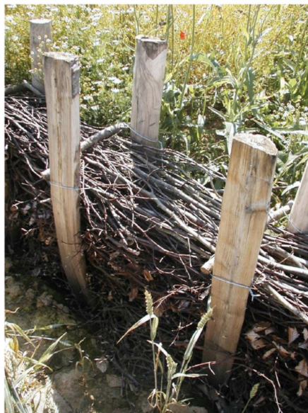
Figure 8. Fascine implanted in the field across the thalweg (Richet et al. 2017).
