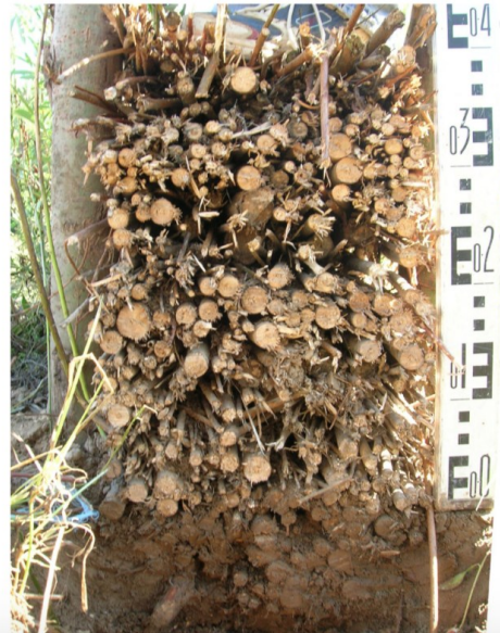
Figure 8. Fascine implanted in the field across the thalweg (Richet et al. 2017).
