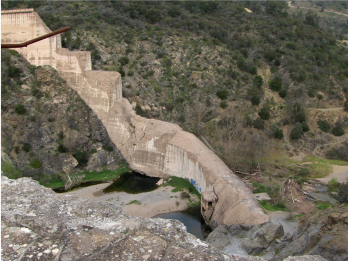
Figure 6.2: Failure of the Malpasset Dam (France) in 1959 - Photos Irstea
