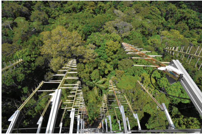
Fig. 2. Twenty antennas installed on the Guyaflux tower
