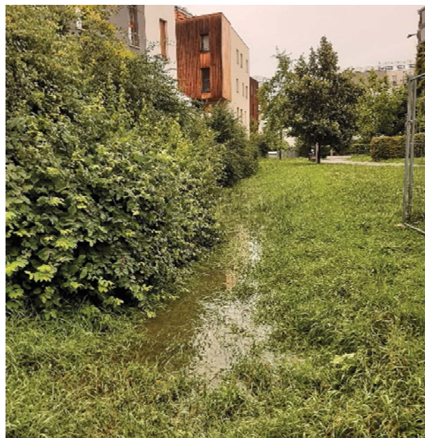
Figure E 2. Infiltration trench in summer 2021.
