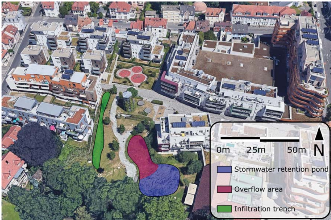
Figure 3. 1. Aerial overview of the investigated field site with the stormwater infiltration pond (blue), overflow area (red) and the infiltration trench (green).
