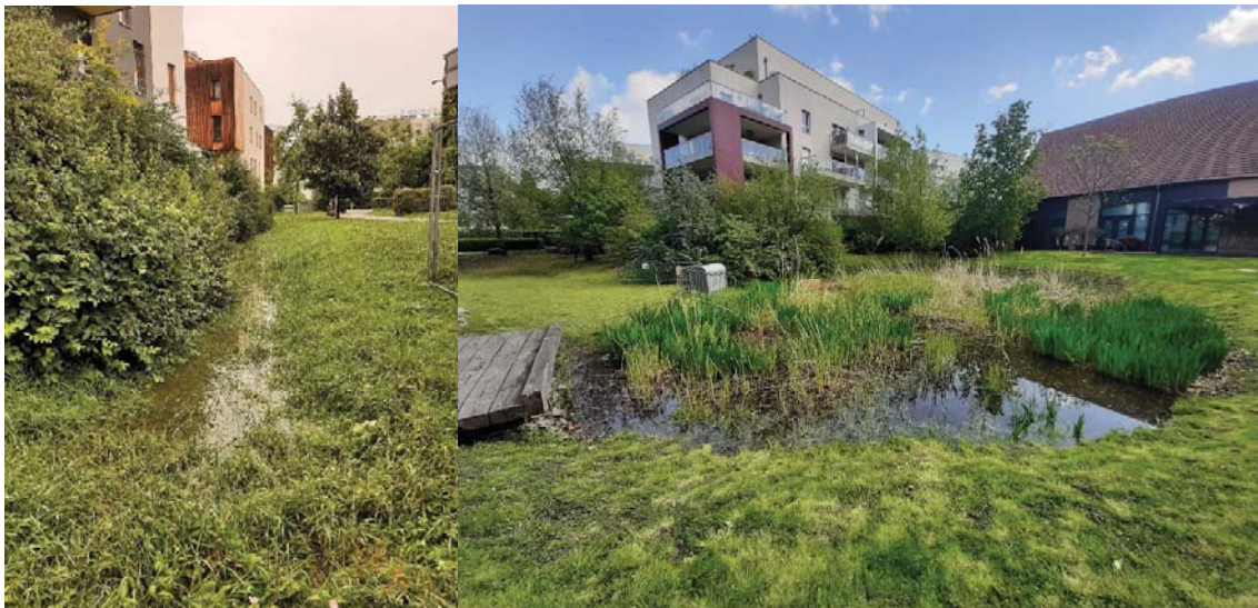
Figure 3. 2. Infiltration trench (left) and vegetated stormwater infiltration pond (right).
