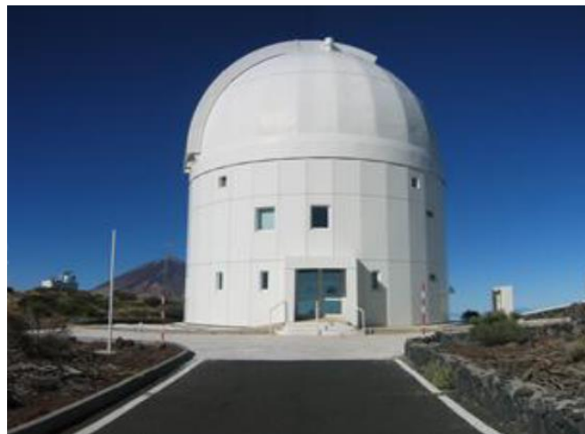
Figure 1-5 : ESA's optical ground station building in Tenerife
