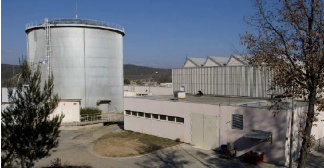
Figure 1.1: MASURCA reactor buildings
