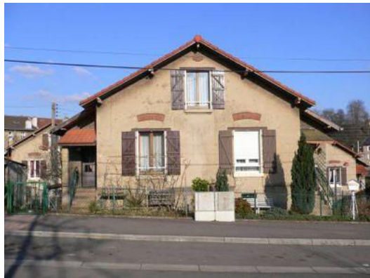
Unreinforced masonry building in zone 3
