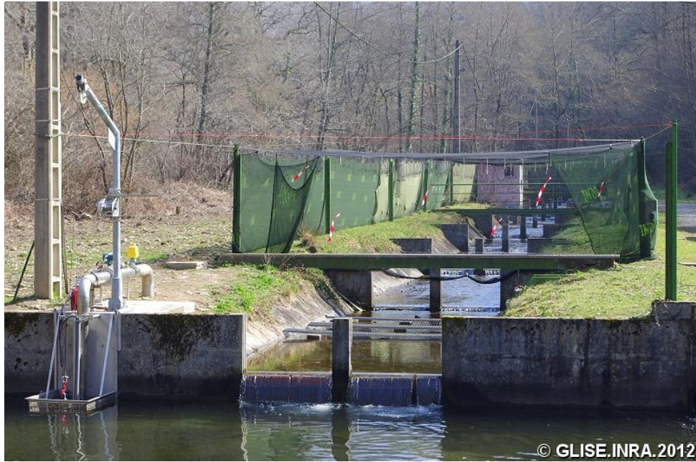
Figure 1. Lapiduxuri experimental channel. Nets are deployed to prevent birds from fishing. Passage between sections can be prevented if required. Substratum can be modified, as well as water depth and shelters availability. Additionally, water discharge can be controlled by tuning the in-flow from the natural river, independently for sections 2 to 7 and 8 to 13 respectively (thanks to a by-pass) and can also be regulated using a water pump (lower left corner of the picture).
