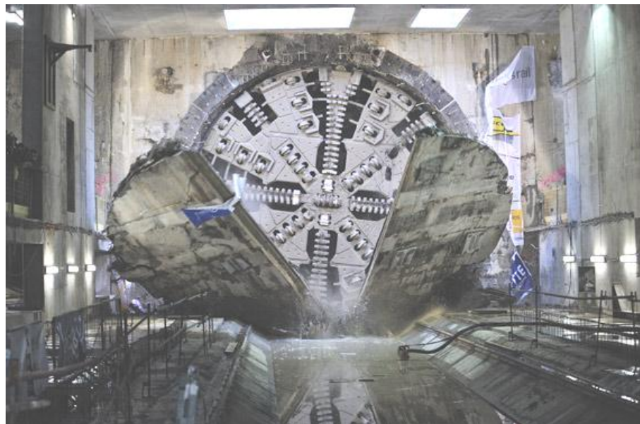
Figure 4-13. TBM arrival to the exit shaft
