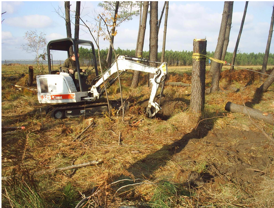
Figure 3.2. A mechanical trencher used during the trenching tests in France.
