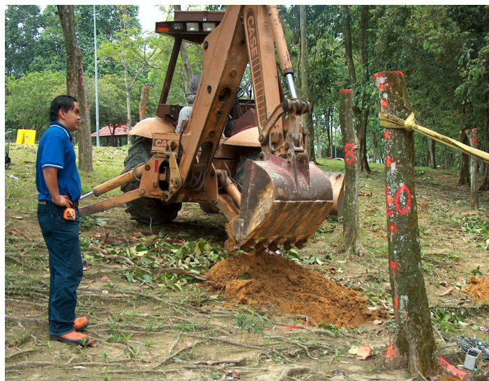
Figure 2.4. A mechanical trencher used during the trenching tests in Malaysia.
